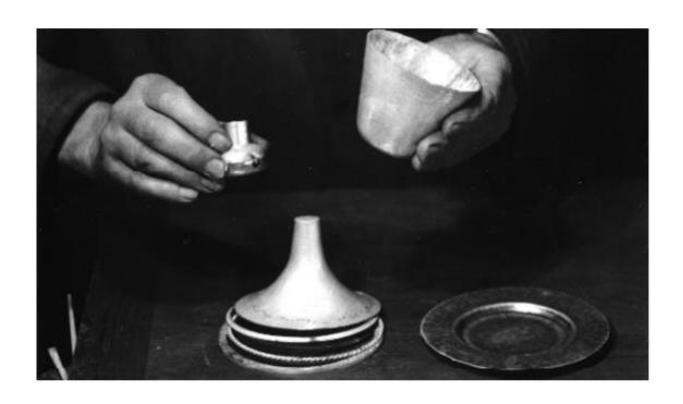
All the parts are now ready to be joined together. The decoration of the base consists of two rectangular wire rings, one twisted wire ring, a trumpet shaped stem and a knop.
