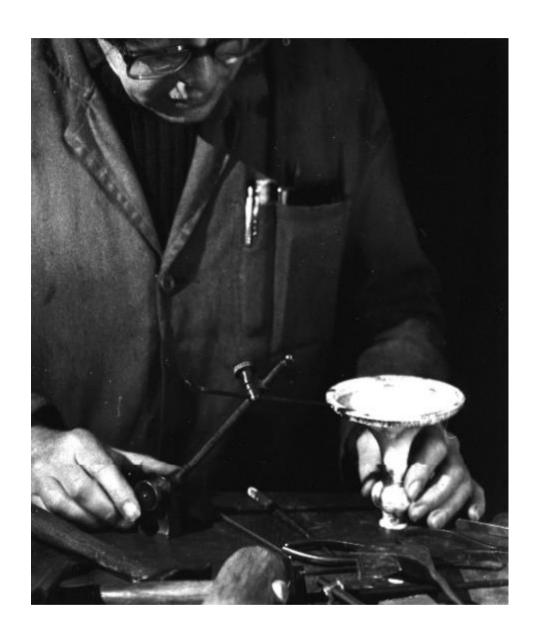
When the knop has been soldered to the stem, the foot is set up on the surface plate to check everything is level.
